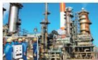
Refinery turbine lubricating oil (SRC-814-15V; explosion proof)
